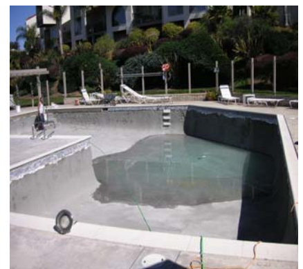
Resurfacing of the pool is underway.
